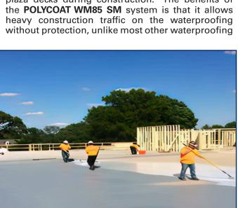
systems and can be installed while construction continues. Additionally, to improve the project schedule, **POLYCOAT WM30 SM** was applied to a third floor deck so that fit out of the apartments units below could begin.
