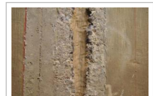
Figure 8 Re-application of joint sealant
