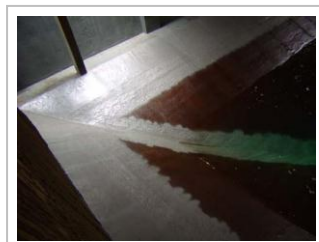
Figures 9, 10, 11 & 12 - Coating of expansion joints, cracks and tank separation walls
