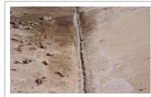
Figure 7 Removal of existing joint sealant
