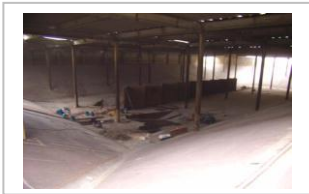
Figure 5 Tank during structural repairs
